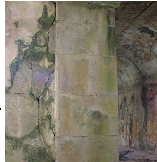
Internal wall of the West wing
