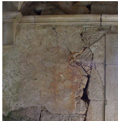
External wall of East wing
