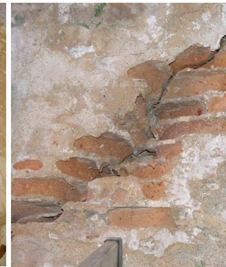
Deterioration of bricks
