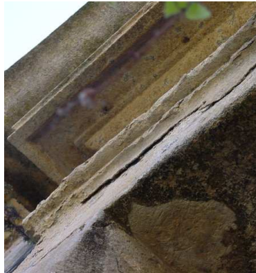
Stone deterioration
