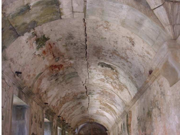
South wing at the 2 nd level
