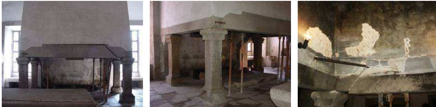
Aspects chimney: In plan size of 4.3 x 4.1 m 2 and 16.2 m height
