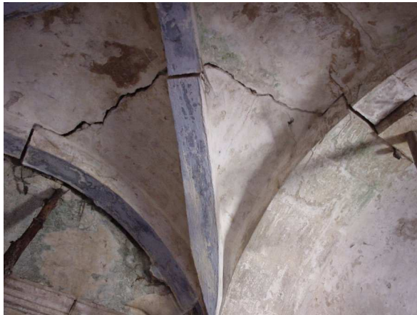
South-West corner at the 2 nd level
