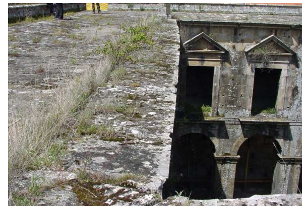
Out of plumbness of walls (2 nd level). Resulted in vertical displacements in vaults' extrados up to 0.10 m
