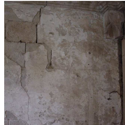
External wall of South wing
