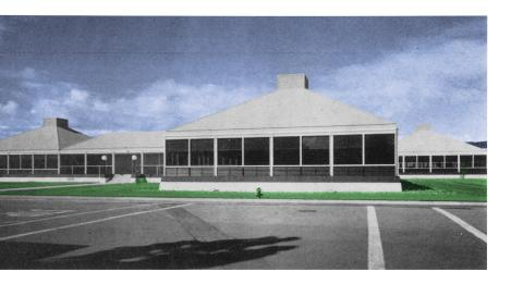
This siting of an extract fan (open to the air) at the apex of a pyramid roof with sound extenuator box beneath represents a neat method of artificially ventilating a square wide-span building.
